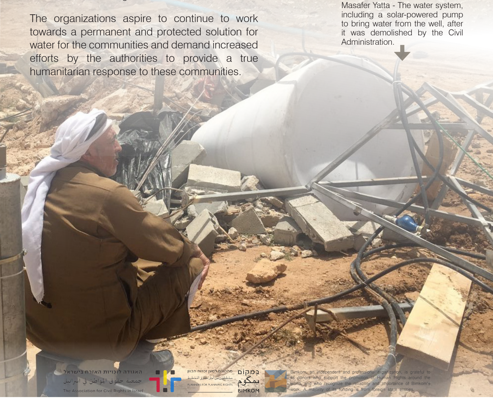
↑ Ghawalliya - a boy next to the only water pipe of the village, minutes after it was cut and disconnected by the Civil Administration.
